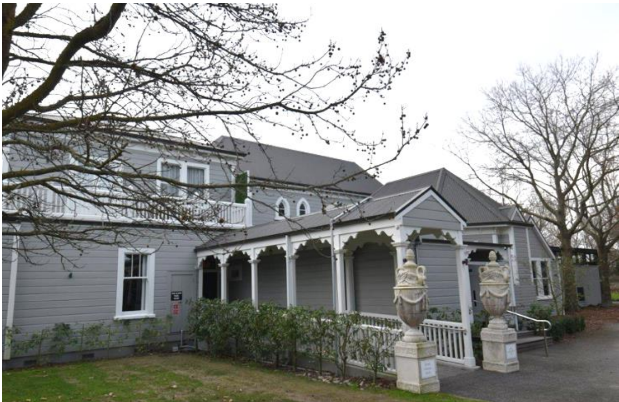
Fig 17: the southern elevation showing additions and extensions, L-R: 2016 reception lounge extension; entrance ramp and canopy; 2016 kitchen infill addition; 2008 'billiards room' addition; 2020 annexe addition; 2020 restaurant addition.
