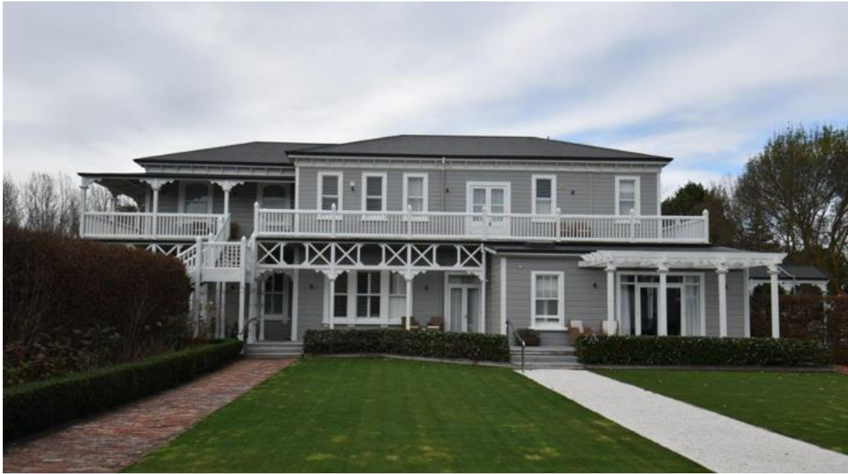
Fig 16: The western elevation showing extended balconies, added external stairs, and extensions and alterations to the upper and lower storeys.
