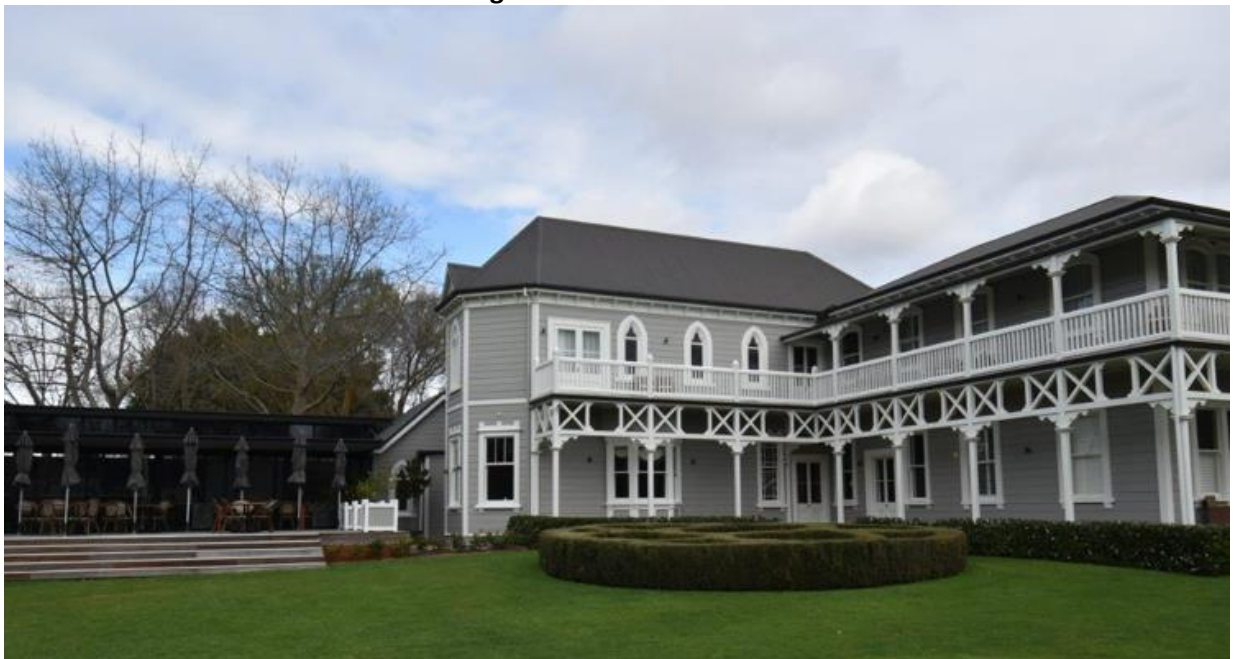
Fig 15: Northern elevation, L-R: The 2020 restaurant addition; the 1909 chapel wing with reconstructed second storey; the 1902 original wing with reconstructed balcony.
