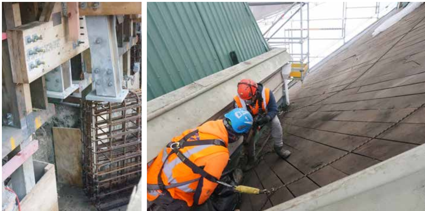
Figure 12: Wesley Church, Wellington (Category 1, List # 4422) – earthquake strengthening and re-roofing 2019-2021 Photo credit: Wesley Church, Paul Cummack, December 2019 (foundation), July 2020 (roof)
