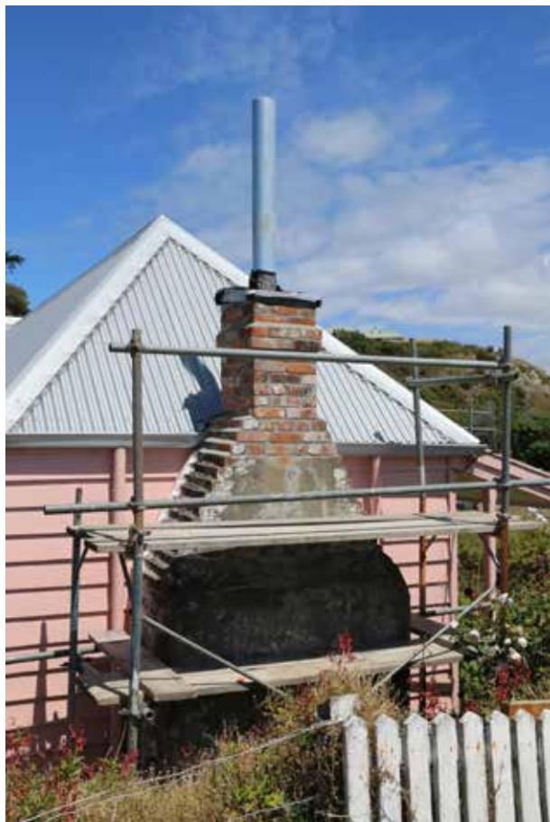
Figure 5: Fyffe House repair and maintenance work: office chimney (showing cement render) and parlour ceiling repairs. Photo credit: Heritage New Zealand Pouhere Taonga, December 2019
