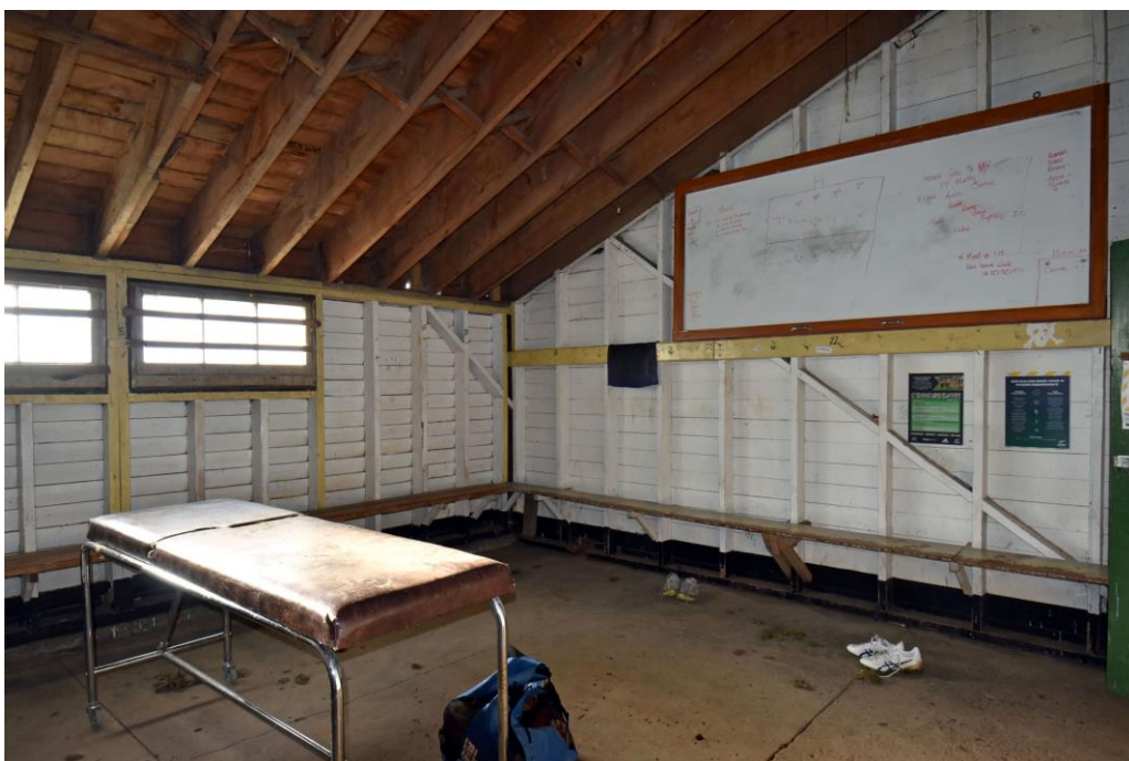
Figure 7: Example changing room underneath the north-western end of the grandstand. Note the original 1924 walls on both visible elevations, Joanna Barnes-Wylie, Heritage New Zealand Pouhere Taonga, 29 April 2022
